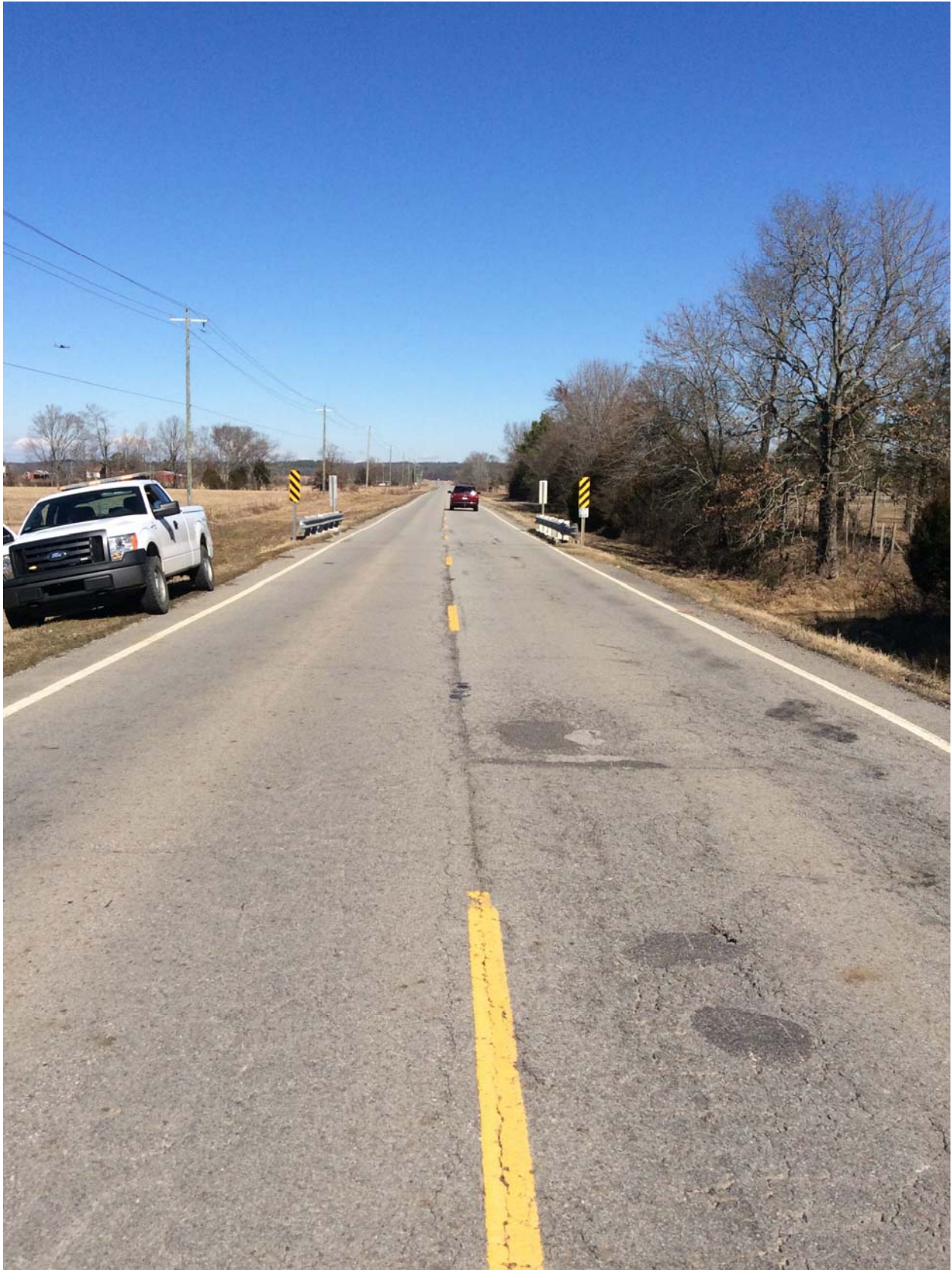
Note: 5.1" of overlay on bridge deck
